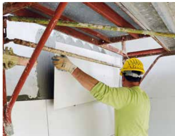
Laying on façades
